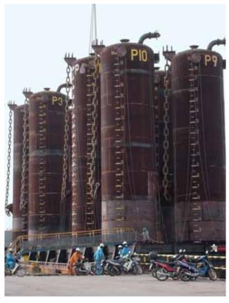
Suction piles for the anchoring of the FPSO Kikeh to be installed by the 'Normand Installer' at a water depth of 1,350 metres
