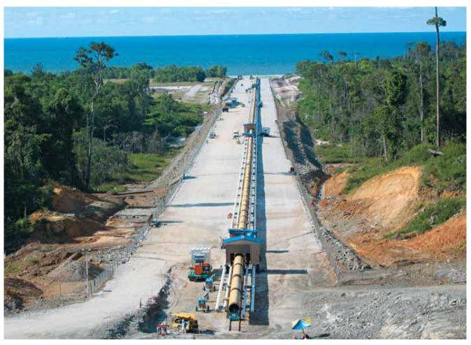
The Gravity Actuated Pipe (GAP<sup>TM</sup>) for the Kikeh field, consisting of a (yellow) carrier pipe and (white) high pressure fluid transfer lines, nearing completion at the assembly and launching site on the coast of Borneo
